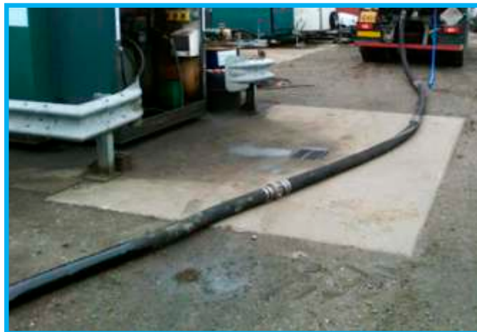
Figure 1. Four hose sections joined together in a vacuum tanker operation with an OhmGuard® hose tester testing the first hose section (blue cable).
