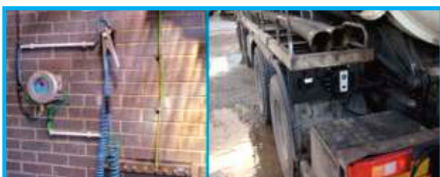
Figure 2: Examples of a gantry mounted (Earth-Rite® RTR) and tanker mounted (Earth-Rite® MGV) static ground verification system.
