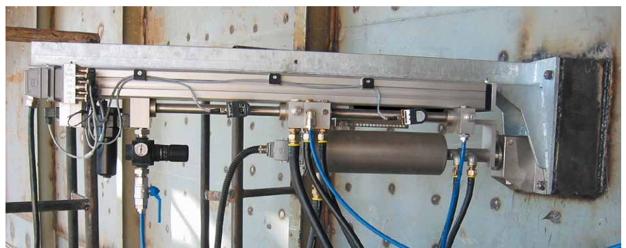
Combustion chamber sensor with retraction unit (water-cooled)
